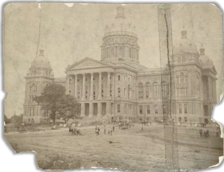
Crews grading Iowa State Capitol grounds. ca 1891
